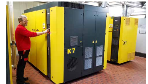
In our Thüringen plant in Austria, we upgraded the compressed air generation with state-of-the-art technology. This led to large savings in electricity and gas (by heat recovery).
